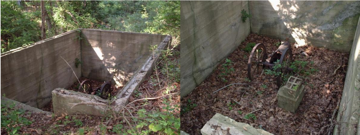
Remains of the pump house (7/14/09)
