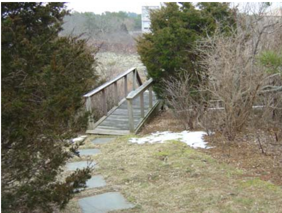
Access from south side of structure to Seabreeze Lane
